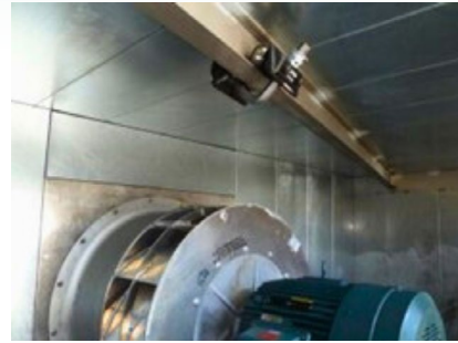
Motor Removal System
