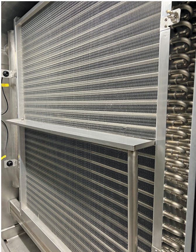
Stainless Steel Tube, Aluminum Fin Evaporator Coil
