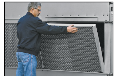
Framed Inlet Louver Design
