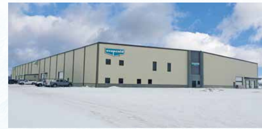
Evapcold Manufacturing, Greenup, IL
