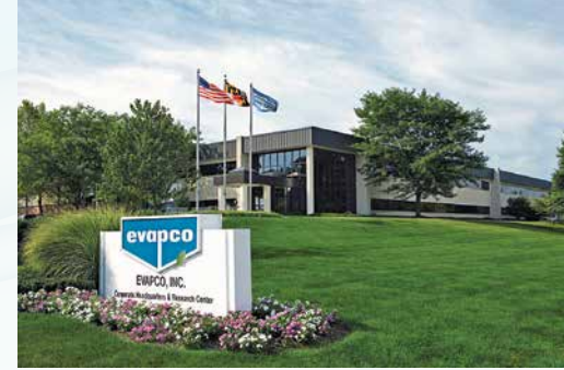
EVAPCO Global Headquarters, Taneytown, Maryland USA
