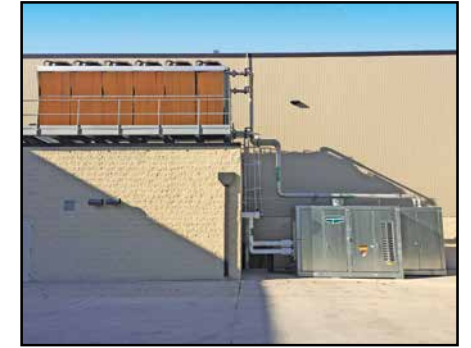
Outdoor manufacturing plant application with enclosure and adiabatic cooler
