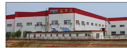
EVAPCO (Beijing) Refrigeration Equipment Co., Ltd, Beijing, China
