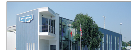
EVAPCO Europe, S.r.l., Milano, Italy
