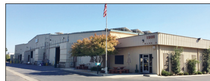
EVAPCO West, Madera, California
