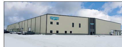
Evapcold Manufacturing, Greenup, Illinois
