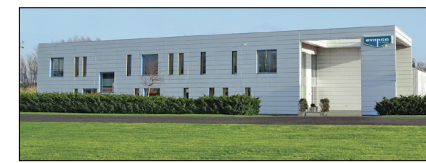
EVAPCO Europe A/S, Aabybro, Denmark
