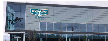
EVAPCO LMP, Laval, Quebec
