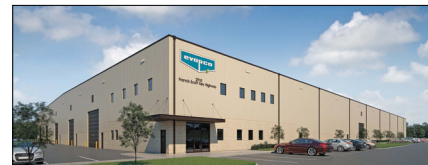
EVAPCO Key Building, Taneytown, Maryland
