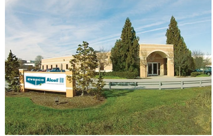
EVAPCO Alcoil, York, Pennsylvania
