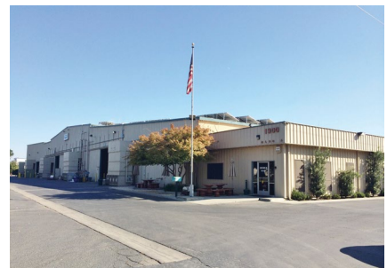
EVAPCO West, Madera, California
