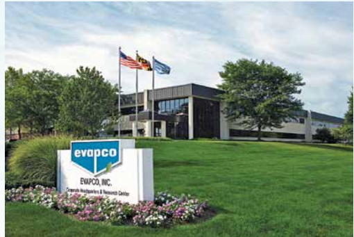
EVAPCO Global Headquarters, Taneytown, Maryland USA
