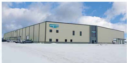
Evapcold Manufacturing, Greenup, IL
