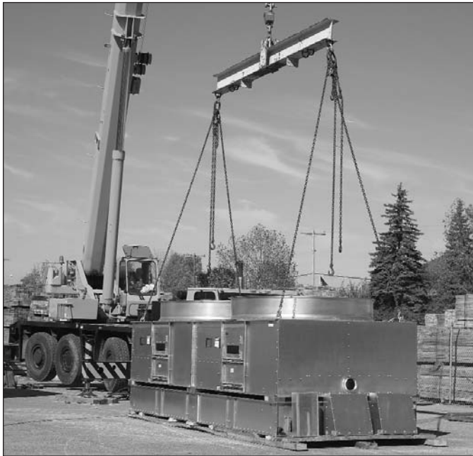
Figure 5 – Lifting arrangement for fan section
