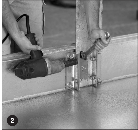
Step #2: Install louver vertical support and tighten hardware.
