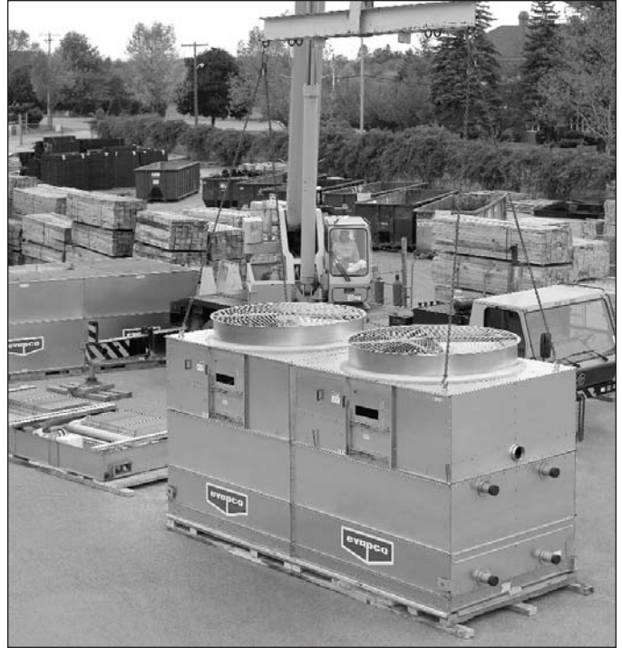
Figure 11 – Assembled fan/coil section
