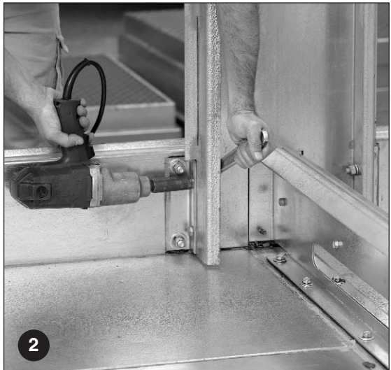
Step #2: Install vertical support and tighten hardware.
