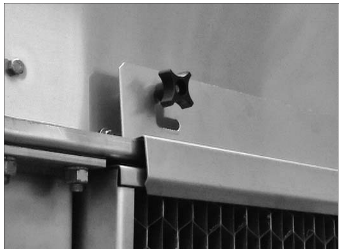
Figure 23 – Installed WST louver
