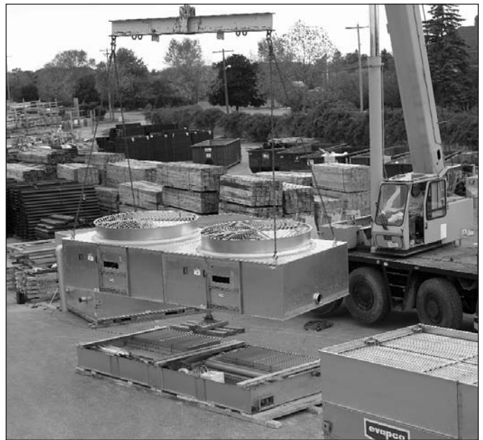
Figure 9 – Lifting of fan section
