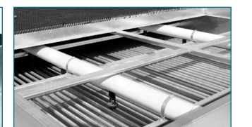
Drift Eliminators Removed for Coil Inspection
