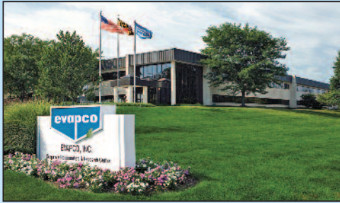
EVAPCO Global Headquarters, Taneytown, Maryland USA
