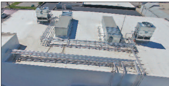
LCR units shown with condenser water piping from fluid cooler (additional roof piping shown serves a separate system)
