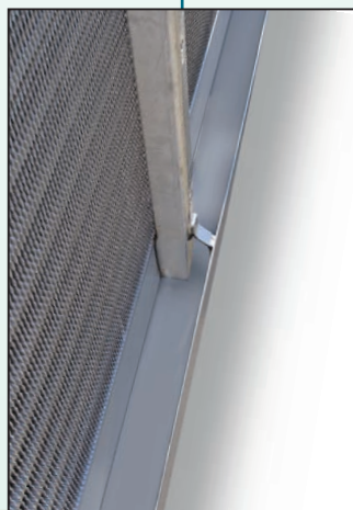
Fully welded pan hanger brackets.
