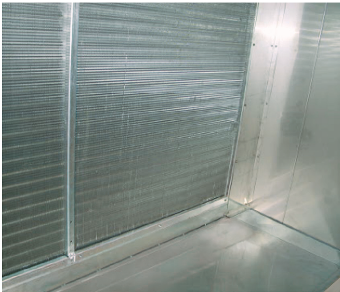
Stainless Steel Tube, Aluminum Fin Evaporator Coil
